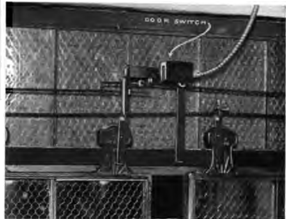
Fig. 4. Electric Door Switch. This insures doors being closed before car leaves landing.
